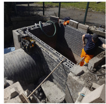
Inspection chamber under construction
