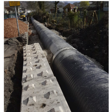
Culvert installation
