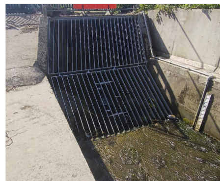
New trash screen at Rhydfach Lower
