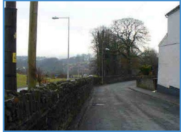
Roadside wall on Forest Road
