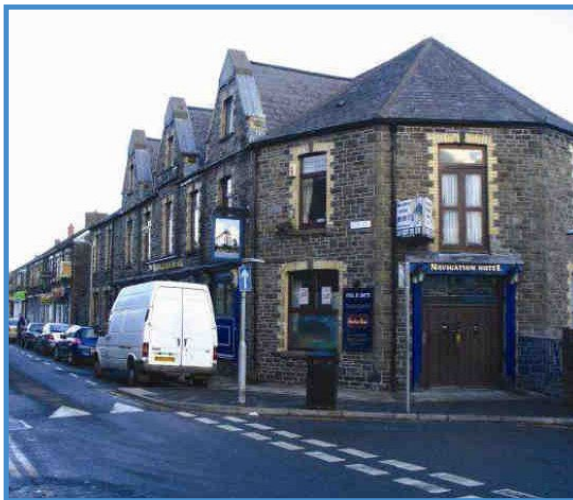
The Navigation Hotel at the entrance to Fox Street settlement.
