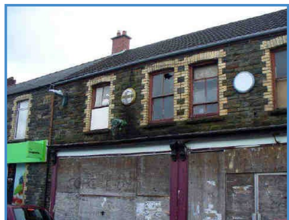
Architectural features remain amidst building conditions
