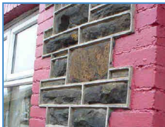
Snecked sandstone masonry
