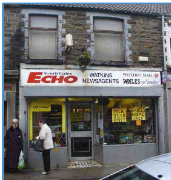
Modern shop fronts fail to reflect architectural details
