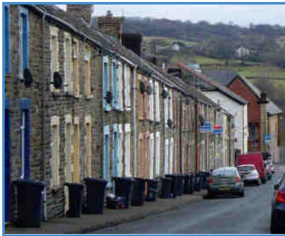
Wheelie bins and satellite dishes detract from appearance
