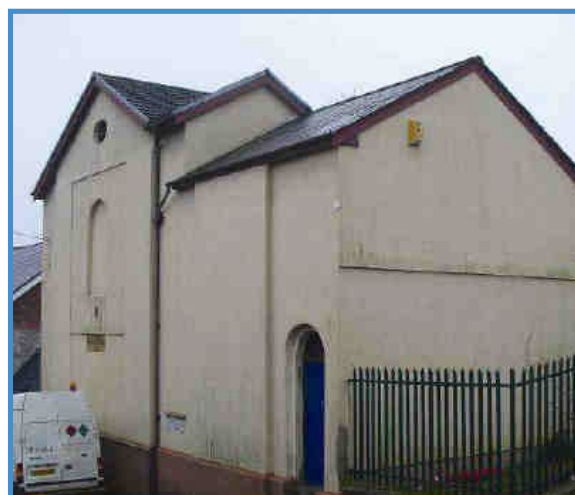
The former Masonic Temple has lost much of its detailing
