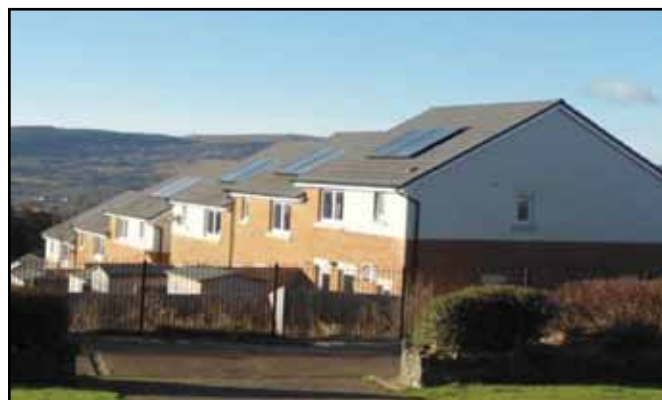
Figure 5.1 Roof mounted solar thermal panels on residential dwellings at Glanmor Gardens, Dowlais.
