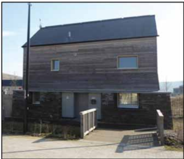
Figure 8.1 Pembrokeshire larch cladding used on the Larch House, the Works Site, Ebbw Vale.
