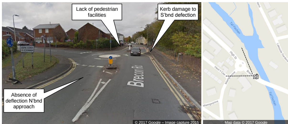
Figure 1 – Maesgwynne Mini-Roundabout Junction – Looking north from Brecon Road towards High Street
