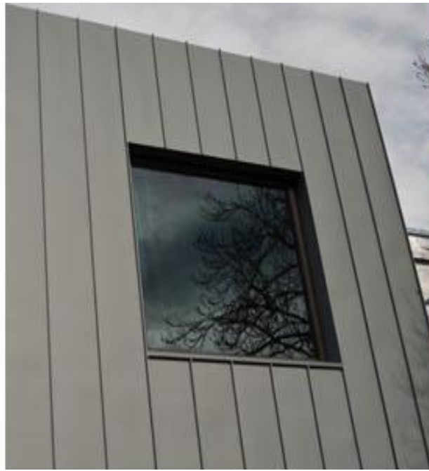
3. Standing Seam zinc cladding to entrance porch
