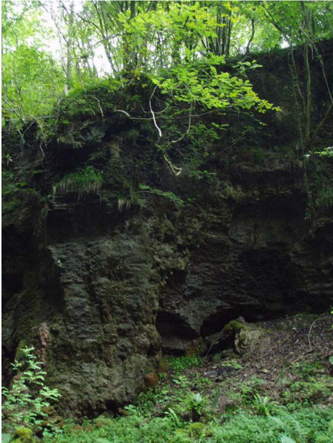
The sides of the Nant Ffrwd gorge are vertical, with loose overhanging sections
