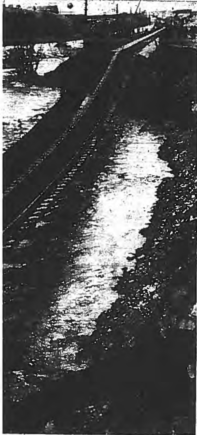
are suspended in mid air after week-end rains. cut the bank and washed away ballast.
