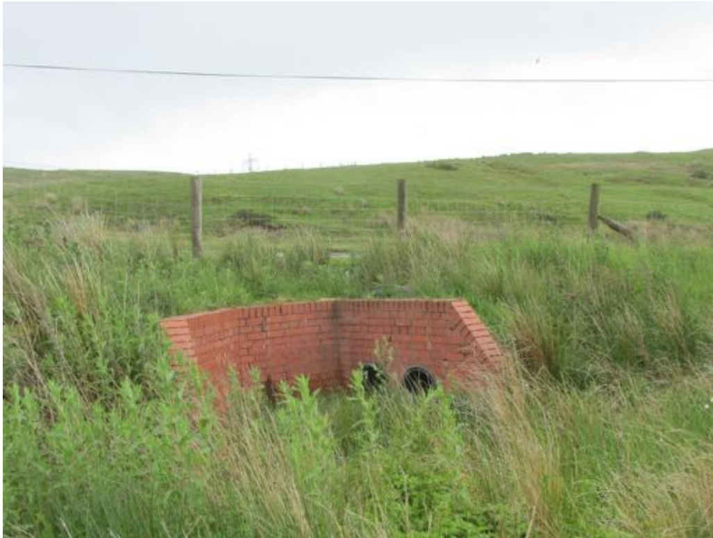
Plate 7. Outfall from wetland back under the Bogey Road
