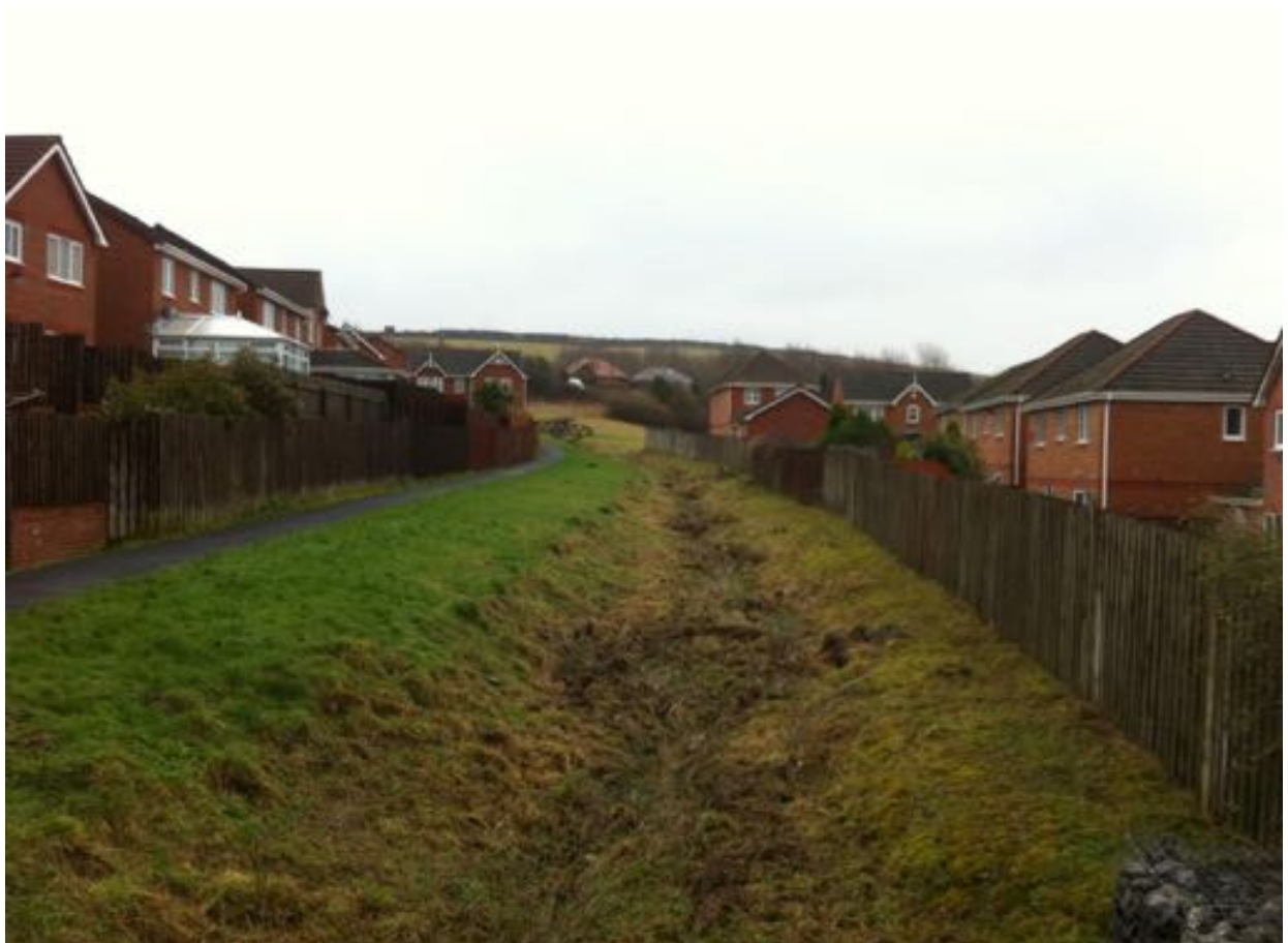
Plate 10. Looking upstream in the Bradley Gardens catchment watercourse at the smallest flow capacity cross section
