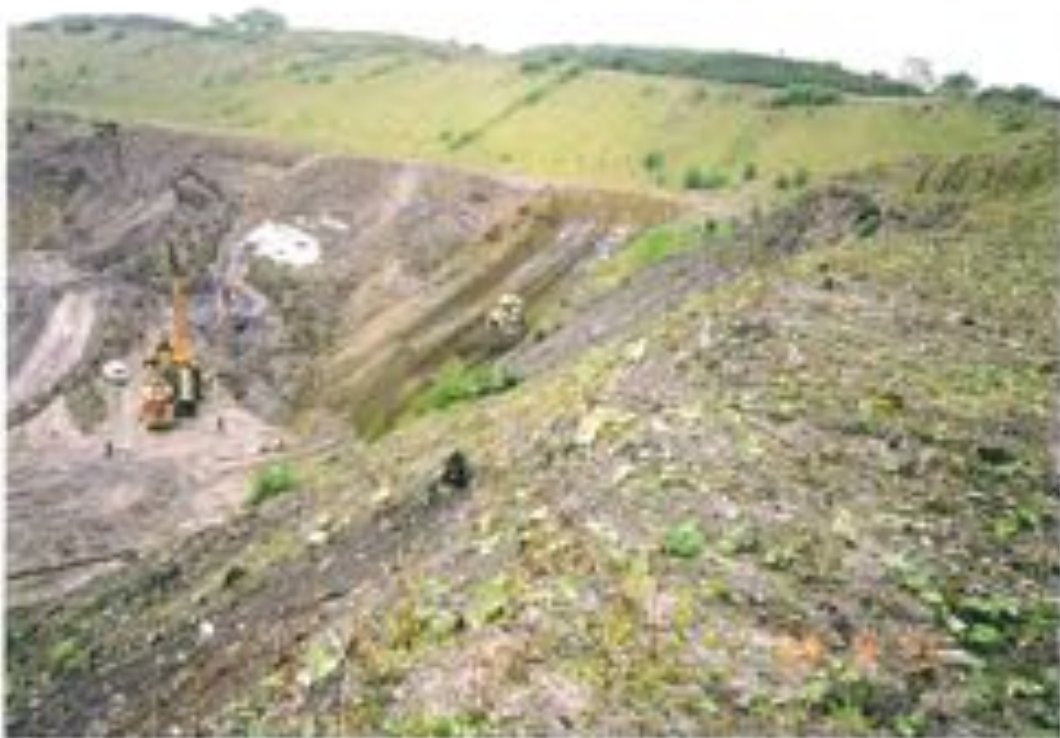
Photograph 21: Example of the successful seeding and natural establishment of vegetation on the drift head batter, significantly reducing its visual impact.
