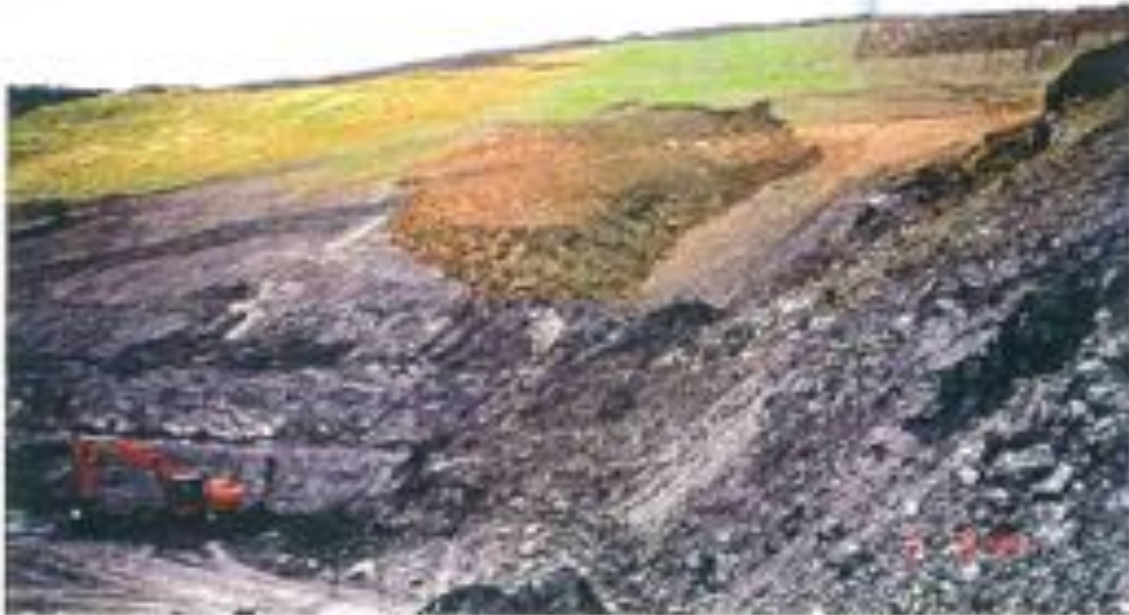
Photograph 20: Example of the temporary seeding of the drift head batter to limit visual intrusion.
