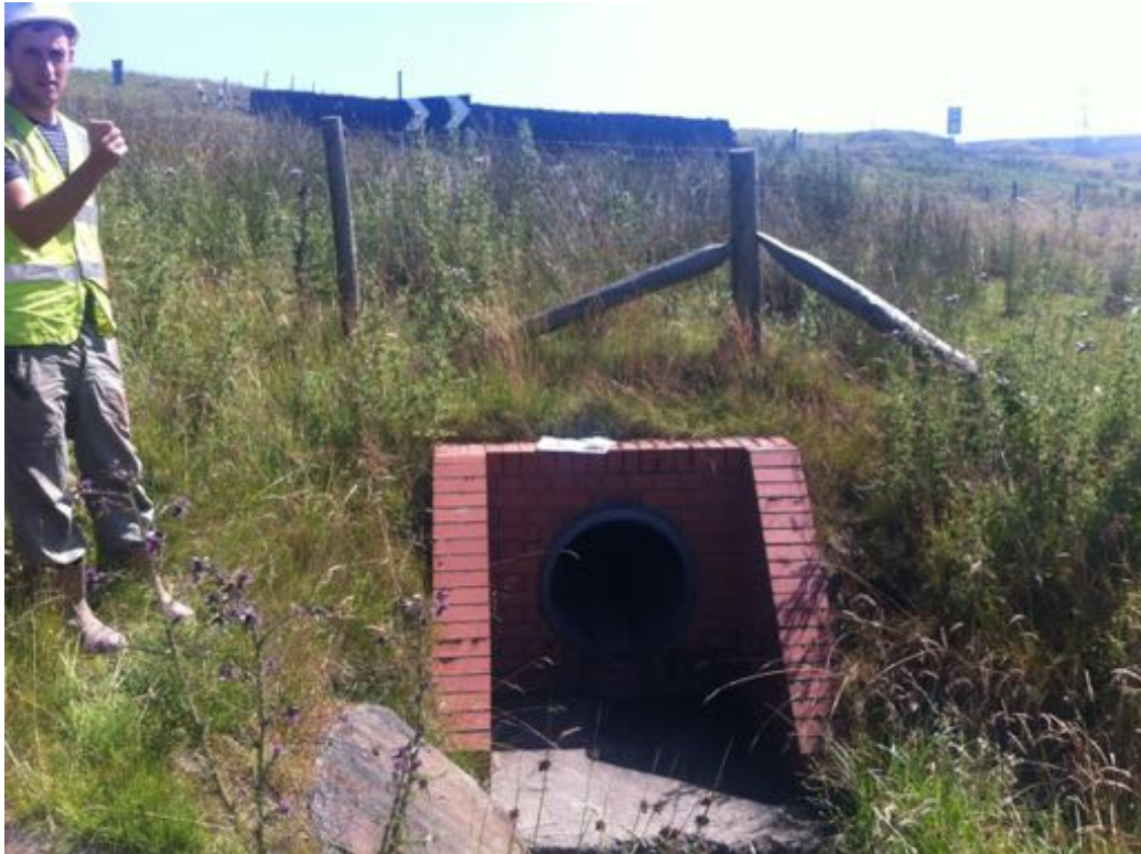
Plate 5. Culvert from under Bogey road draining the railway cutting
