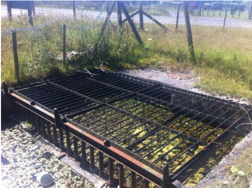
Plate 9. Cwm Blacs A culvert inflow structure
