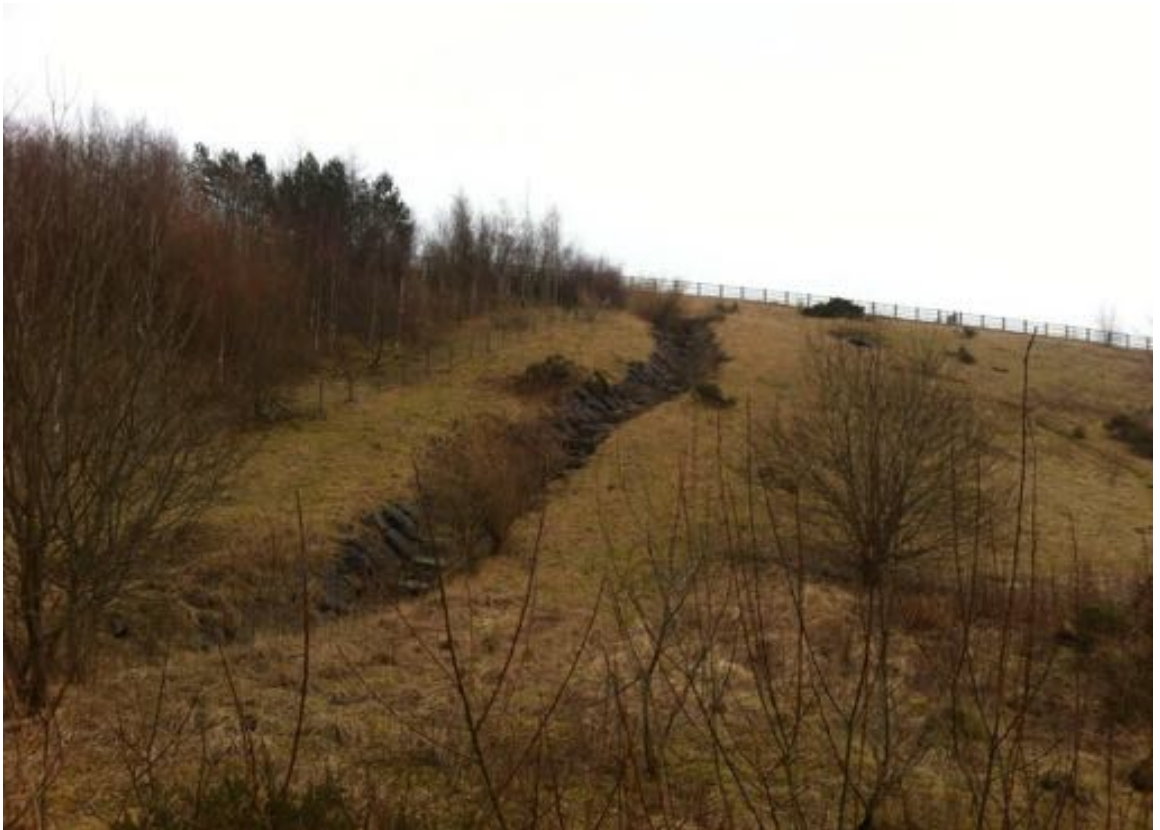
Plate 13. Engineered channel immediately downstream of the Morlais B outfall
