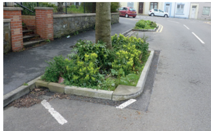
Example - Bioretention system in road build out, Llanelli
